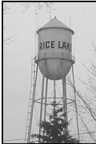
Pictured: Rice Lake Utilities first water tower built in 1925 and still in use today.
